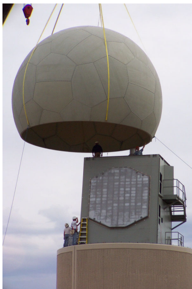
Installation of the SPY-1A antenna and radome on the NWRT
